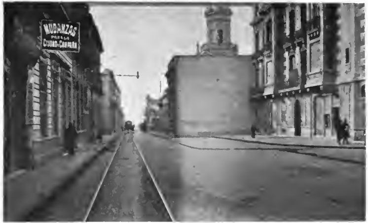
This shows how many of the narrow streets in the older sections of Buenos Aires are being widened. The widening process is carried on generally on one side of the street. The large new building at the right is set back to the new street line with which all the houses on the block will eventually correspond.
